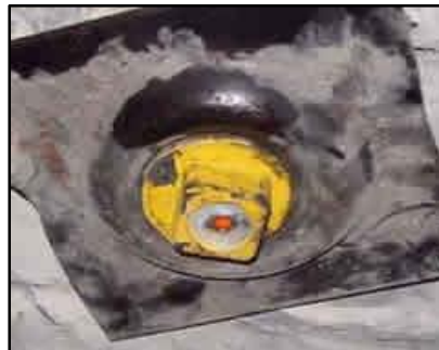
SmartBolt with insufficient tension
